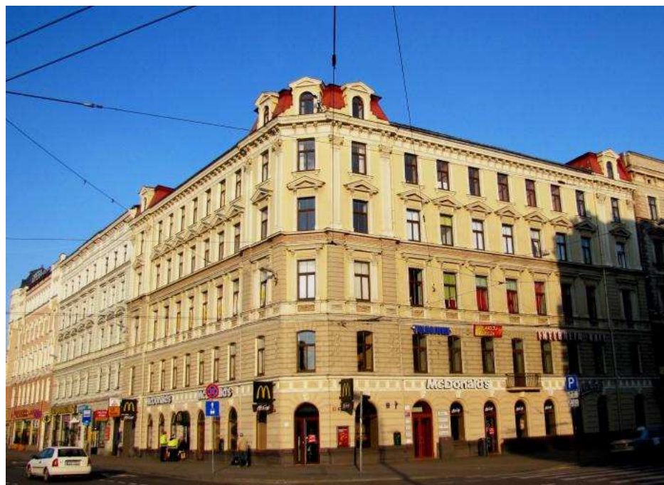
Commercial & office building – Merkela Street, Riga, Latvia
